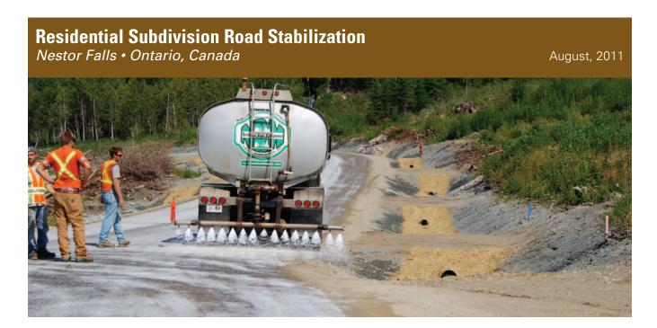
**Project Description:** A newly constructed unpaved residential road was treated with T-PRO® 500 polymer to control fugitive dust emissions.
